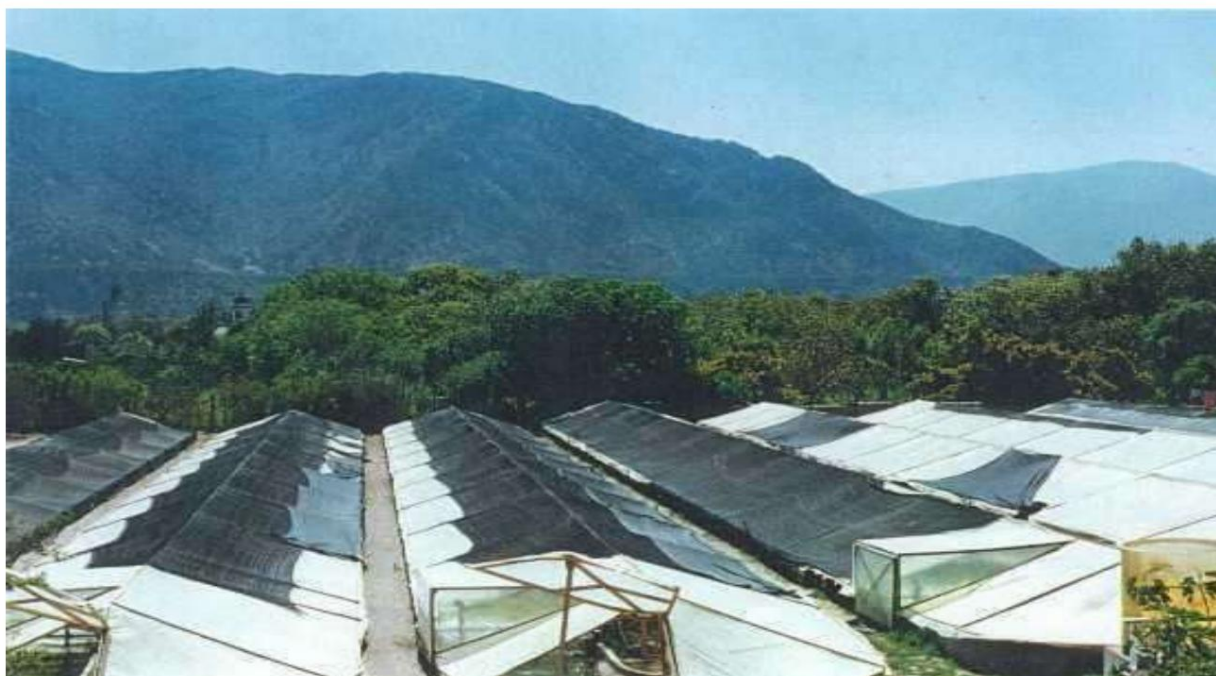
At Bionor, near La Serena, Valle de Elqui (Chile), 1997: only the heads of the basins are made of cement, the rest is made of semi-rigid ethylene-propylene film (end embedded in concrete), the greenhouses have a wooden frame .
